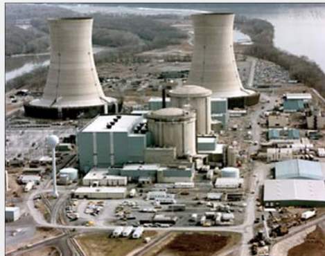
Figure 2: Management at the Three Mile Island nuclear accident showed poor authenticity
